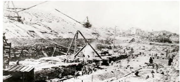
Soo Locks under construction
